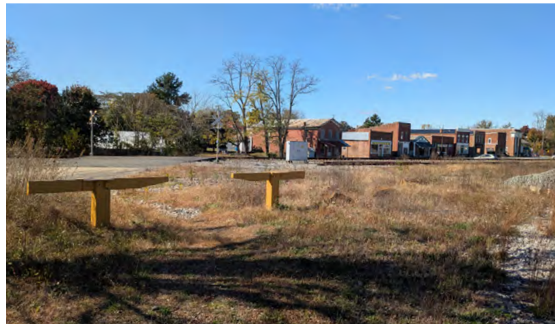
Figure 35 – Existing railroad crossing in the Town of Pamplin City
