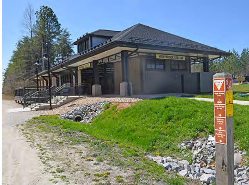
Figure 34 – High Bridge Station Visitor Center
