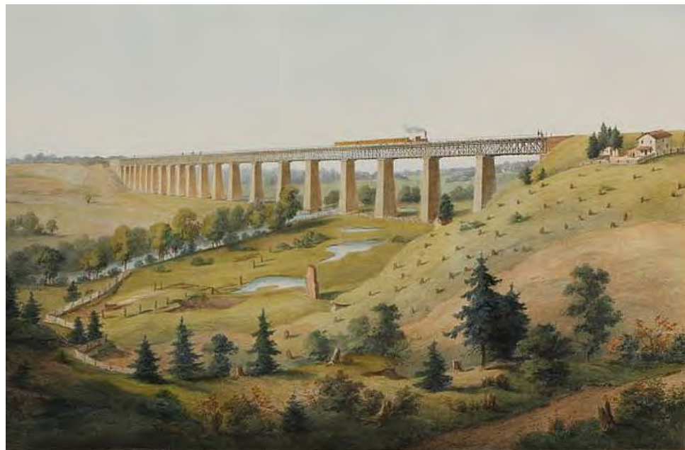
Figure 18 – The original High Bridge spans the Appomattox River east of Farmville in this 1857 lithograph by German artist Edward Beyer
